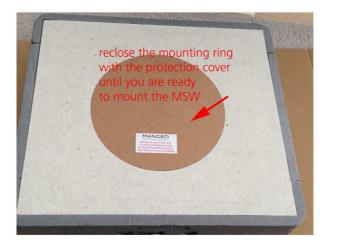
reclose the cabinet with the protection cover finish the wall and fill the gap with silicone sealing
